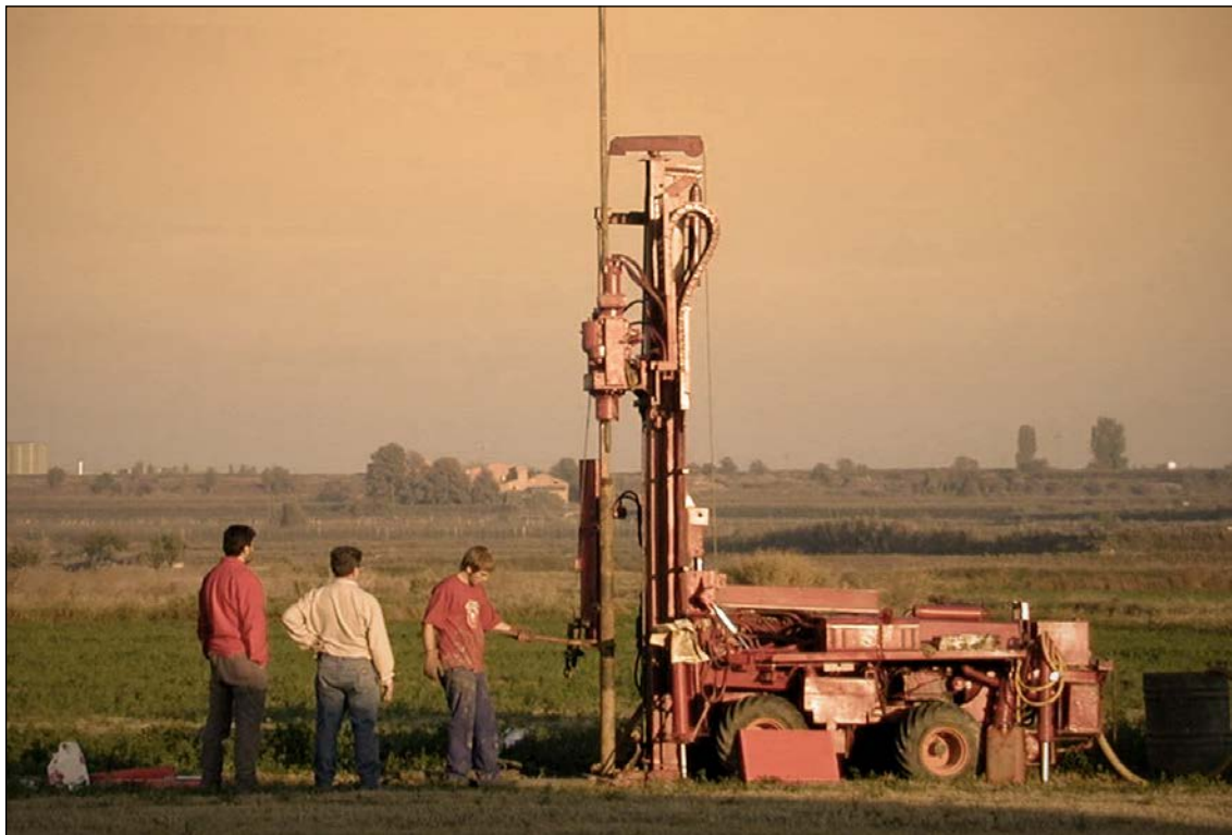
Fig. 53. Hydraulic and mechanical drill operating at Ivars lake before re-filling operations.
