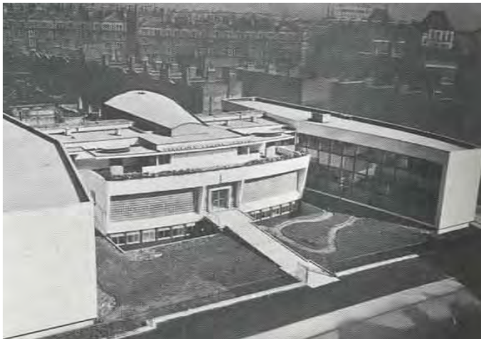
55. Vista general del Finnsbury Health Center. Lubetkin.
