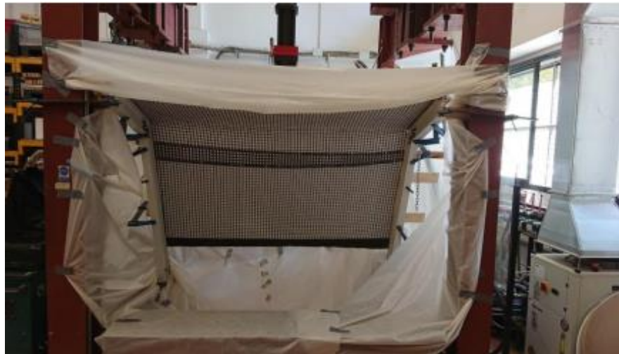
Figure 53. Porexpan plates placed on the fiberglass meshes
