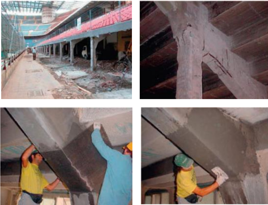
Figure 7. Strengthening San Siro stadium (Chellapandian and Suriya Prakash, 2021)
