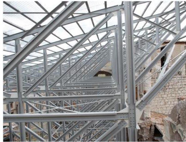
Structural beams (Francesca and Salvatore, 2016)
