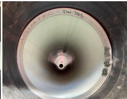
c) Inside view after the rehabilitation
