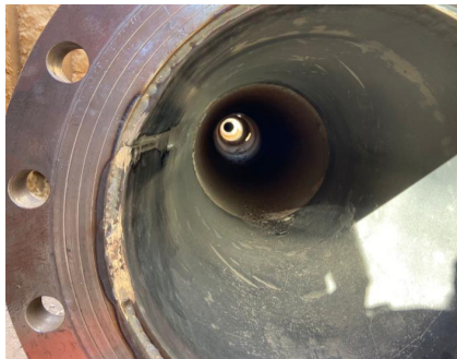
b) Inside view before the rehabilitation
