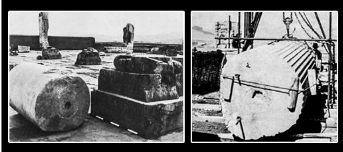
Figure 66: Columns in Pasargad and Persepolis Limited Use of the Anathyrosis Technique for the Construction of Pillars in Pasargadae (Left) and Persepolis (Right) (Motamedmanesh, 2018, p13)
