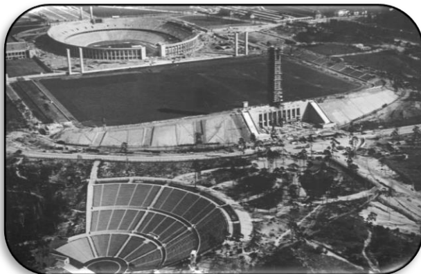
Figure 22 Construction of the Olympic Stadium Berlin 1936 (Source: CC)
