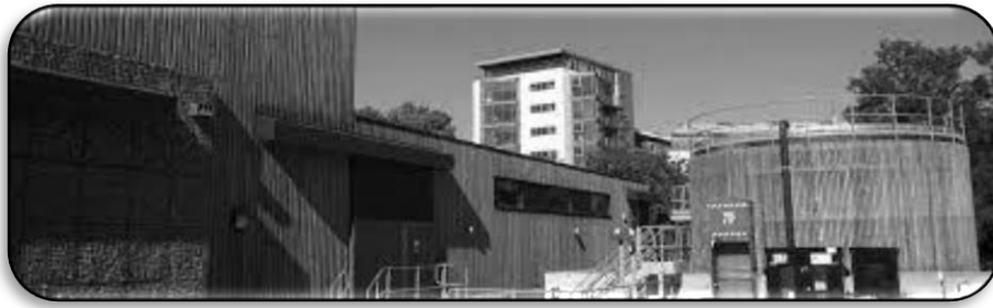
Figure 27 Old Ford factory for wastewater recycling at London 2012 (Source: CC)
