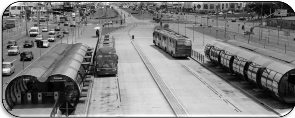
Figure 44 BRT networks in Rio 2016 (Source: CC)
