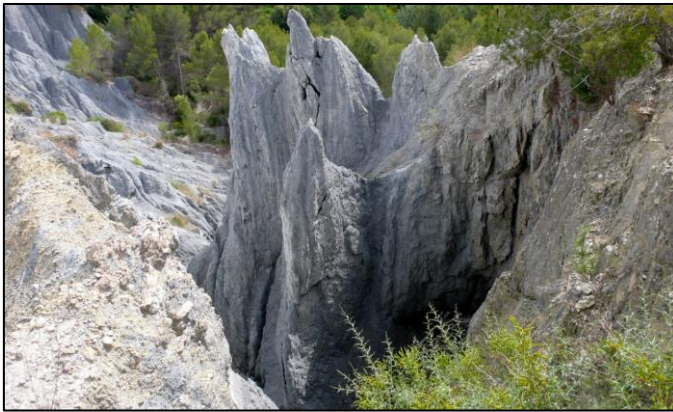
Figure 52. Fault gouge outcrop in Ribes Blaves. This formation is the result of the Paleozoic metamorphic unit affected by the Vallès Fault. Although this formation outcrops far from the study area, it shows an example of the fragile behavior of the metamorphic series in contact with a major fault.
