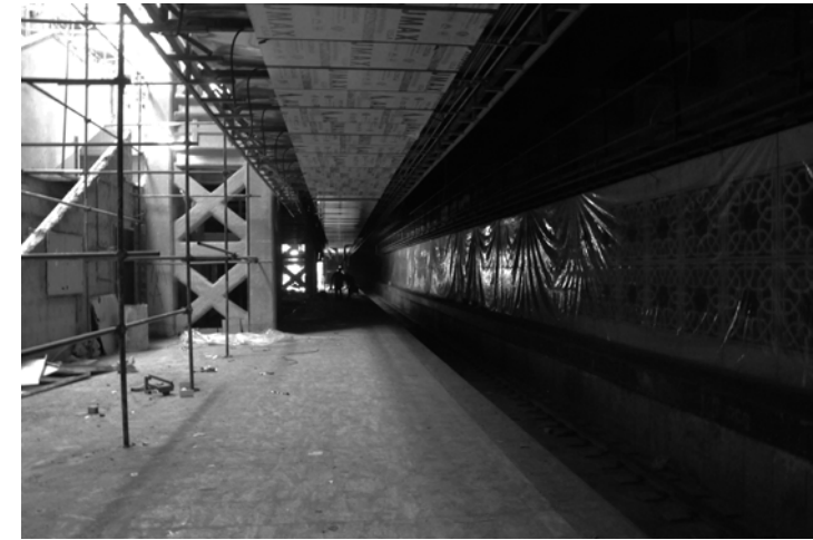
Fig. 336. The under construction eastern side of central platform, February 2016. Source: author
