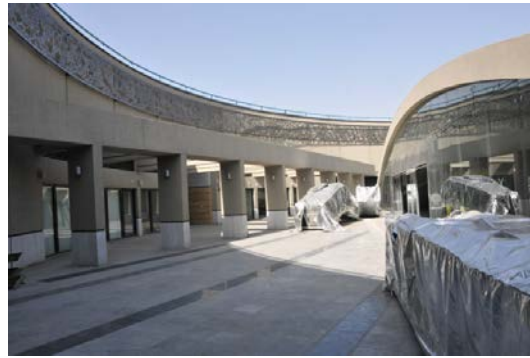
Fig. 350. Commercial units set around the circular central yard, February 2016. Source: author
