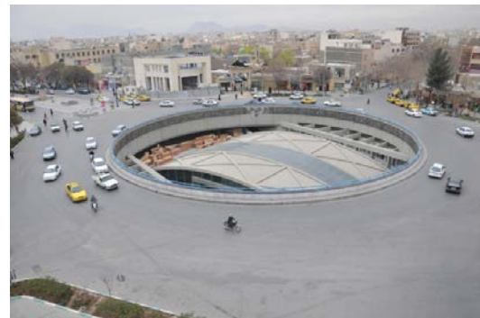
Fig. 342. View from the top of Parto Commercial building to the metro station at the center of Shohada square and the station's entrance at the Square's southwest corner. February 2016. Source: author
