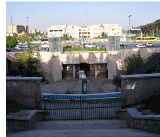
Fig. 291. Defae Moqadas metro station Entrance in front of Kaveh Bus terminal, April 2022. Source: author
