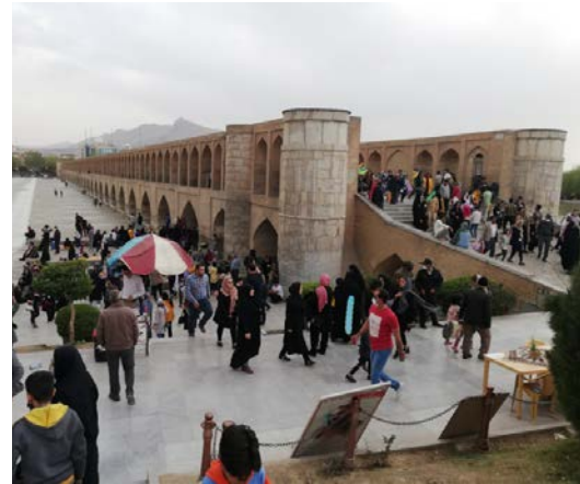
Fig. 145. The north head of Si-o-Se Pol Bridge, April 2022. Source: author
