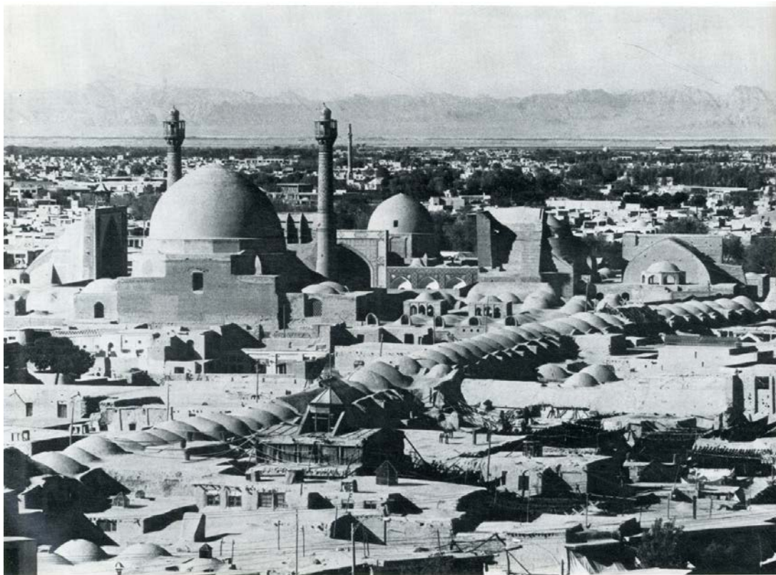
Fig. 49. Looking north towards the Friday Mosque with the bazaar route (foreground) traced by the continuous line of brick domes, Source: The architectural review, Sherban Cantacuzino, 1976.
