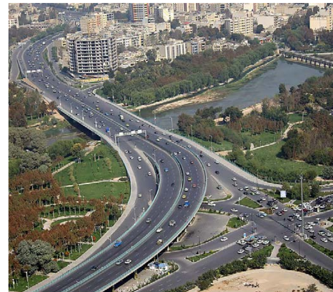
Fig. 212. Frame c, Vahid bridge, the intersection of the Second ring (Khayam expressway) with the river and riverside parks. Source: Atlas of Esfahan metropolis, by Esfahan municipality.
