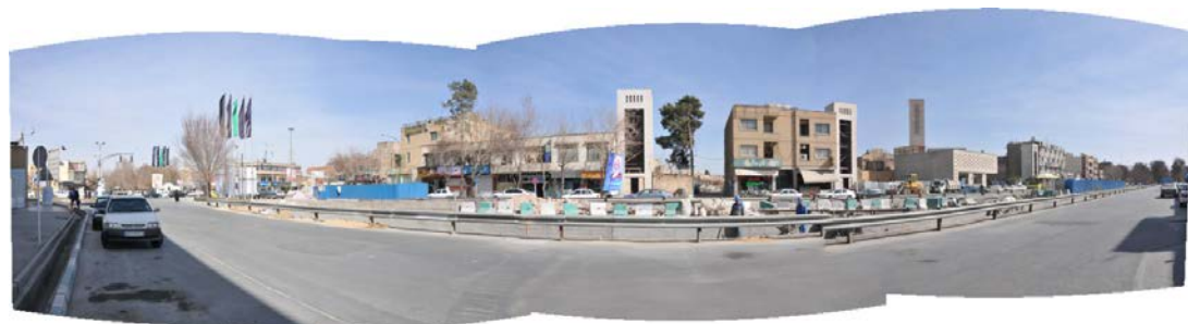
Fig. 334. Takhti metro station circulating towers at the eastern front of the Chahar-Bagh-e-Paieen street, February 2016. Source: author
