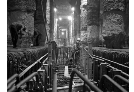
Fig. 294. Metro Line 2 under construction, 2019. Source: Mashreghnews.ir, Mohammad Reza Sharif.
