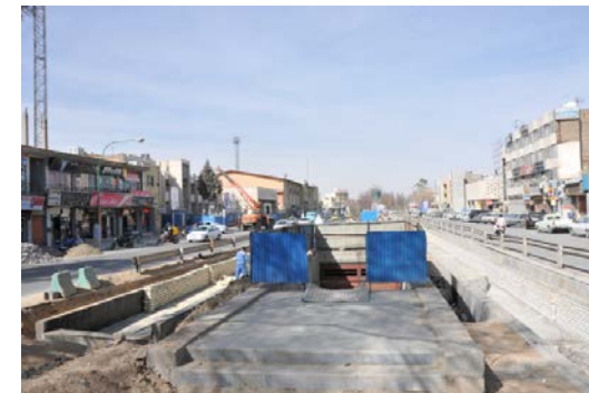
Fig. 338. The Takhti station's southern emergency exit, February 2016, Source: author
