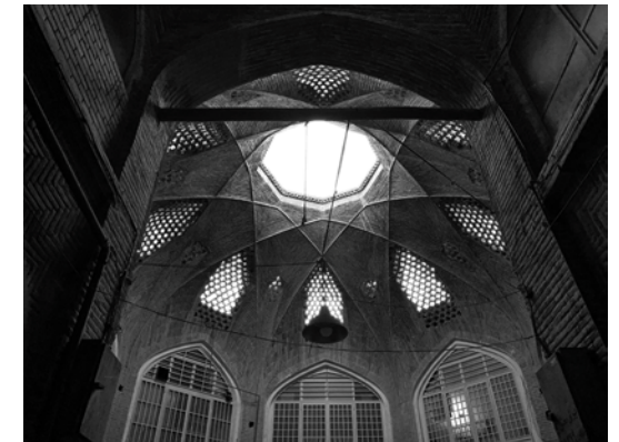
Fig. 81. Se-Rah-e-Nim-Avard_ ceiling of Timche Haj Karim. Photo took by Peyman Baktash, June 2020.
