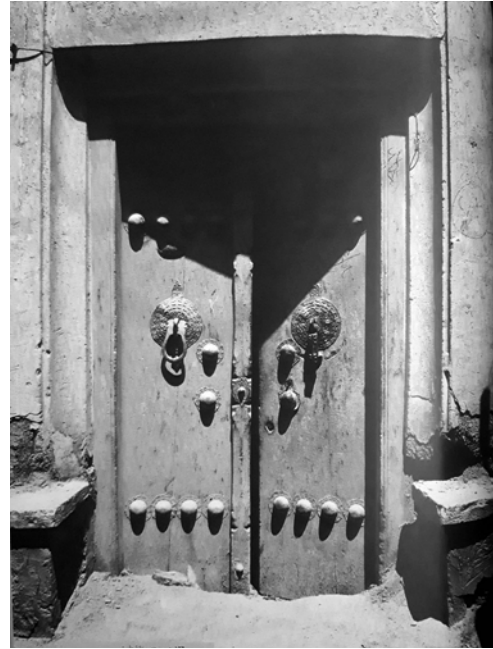
Fig. 121. The main entrance door of Daruiee house, source: Maisons d'Ispahan, Darab Diba.
