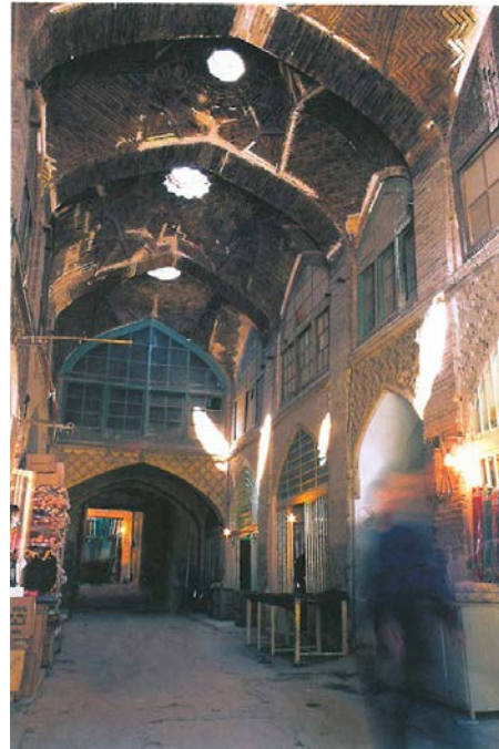
Fig. 58. Northern Dalan of the Sarai-e-Golshan. Source: Ganjnameh: Cyclopaedia of Iranian Islamic Architecture- Vol. 9
