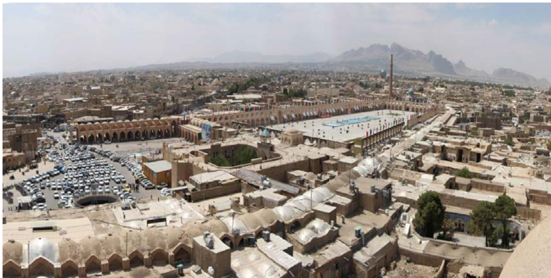
Fig. 255. Perspective of the Atigh Square from the top of Jame Mosque's minaret, 2016. Source: Esfahan municipality.
