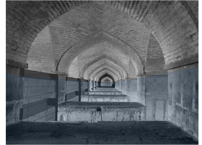
Fig. 155. Sealing the water and creating a dam under the Khaju bridge's arches. Source: https://www.itto.org/iran/image-bin/khaju-bridge-arches.jpg edited by the author
