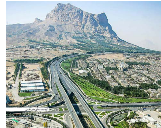
Fig. 211. Frame b, Sofeh mountain, Maidan-e-Defa-e-Moghadas, the intersection of the Second Ring with Hezar-Jirib avenue and Dastjerdi expressway (Shiraz way).
