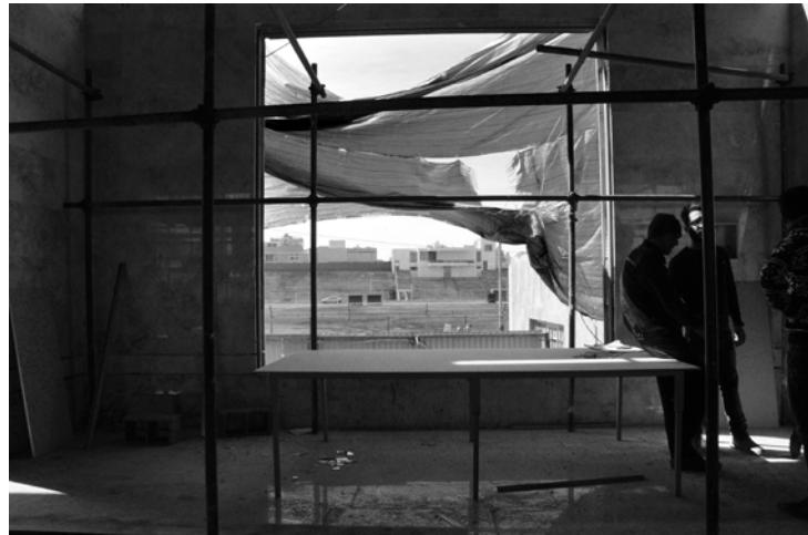
Fig. 330. The view from the western entrance to the stadium, February 2016. Source: author
