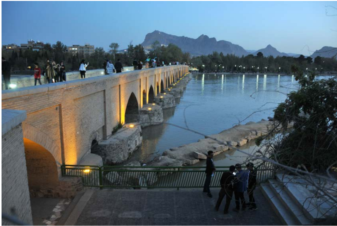
Fig. 142. Marnan Bridge, April 2022. Source: author
