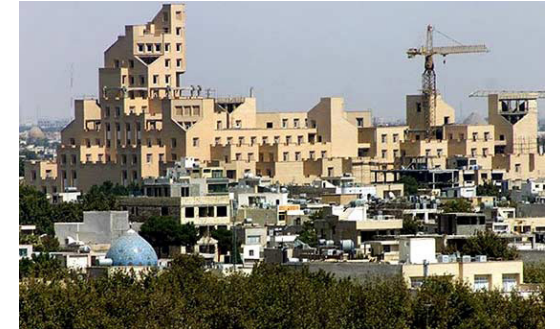
Fig. 314. View to the Jahan Nama tower building from the river side. Source: unknown
