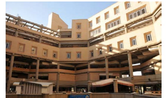
Fig. 315. At the ground floor, inside the patio of Jahan Nama complex center, February 2016. Source: author
