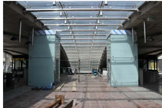
Fig. 352. The arched glass roof enters the skylight to the ticket hall and the central platform levels, February 2016. Source: author
