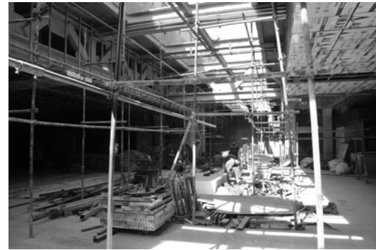
Fig. 333. Takhti Station ticket hall, 2016. Source: author
