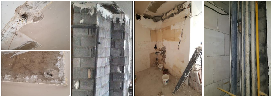
Figure 5.8. Interior and exterior walls of the initial state
