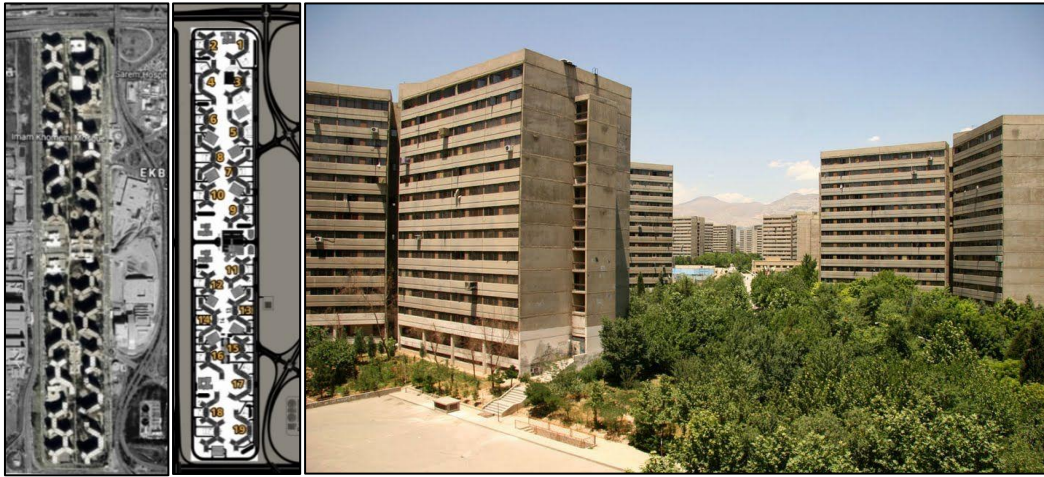
Figure 4.21. Phase-2 of Ekbatan. Source:(left) Author, (right): Safa Daneshvar ( http://safa.daneshvar.ir ).
