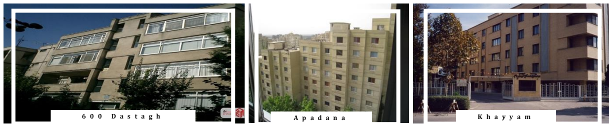
Figure 2.3. MHs constructed in the second period (1960 to 1980)
