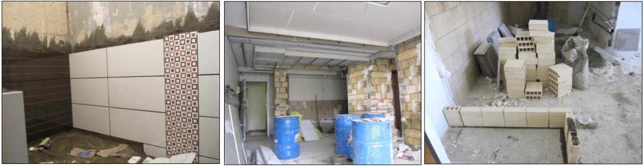
Figure 5.21. Rehabilitation process of scenario 2.
