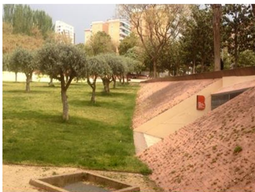
c. Brick slopes
