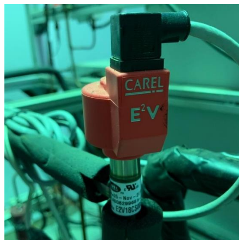
Figure 2.6. E2V18 Back-pressure valve.
