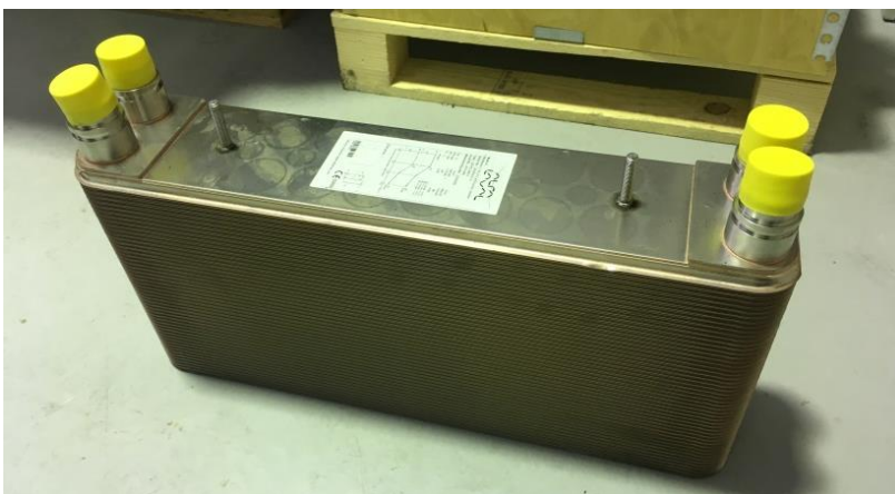
Figure 2.11. Evaporator brazed plate heat exchanger of 4.794 m 2 of exchange surface area.
