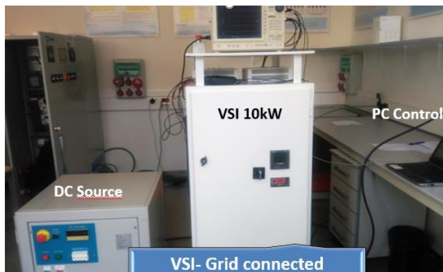
Figure 120: Experimental setup of a 10 kVA power converter.
