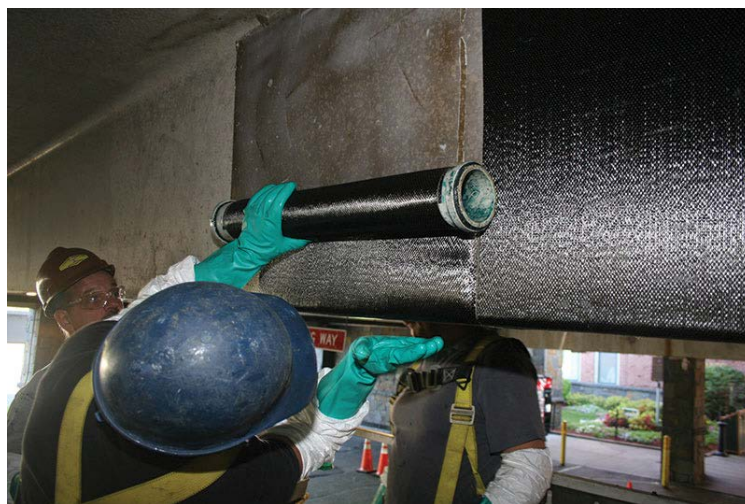
Figure 3. Strengthened structure with FRP (Nystrom et al. 2003).
