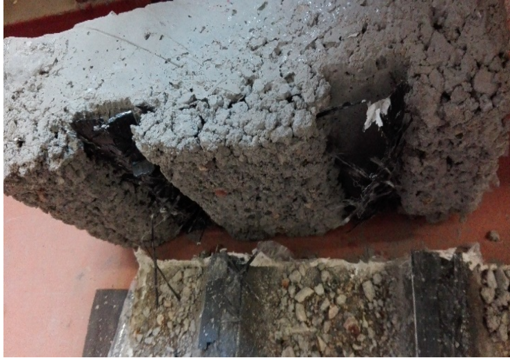
Figure 28. Shear test failure mode.
