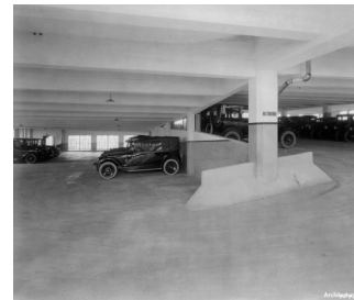
2.1.1-1_Fort Shelby Garage in Detroit-Albert Kahn_1922
