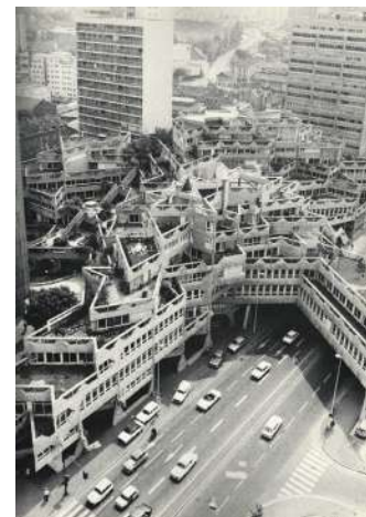
PV.2.4-8_Housing Building-Ivry-sur-Seine_Jean Renaudie-Renée Gailhoustet's_1969-1975
