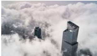
4.3-2_Hitachi elevators-CTF Finance Center-Guangzhou, 2017
