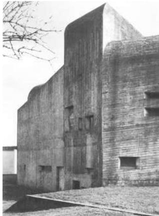
1.3.4.4-1_Detail of the North facade-2004. Nevers_p33
