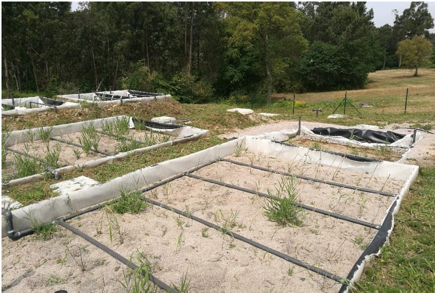
Figure 4.3. Overview of the vertical subsurface flow constructed wetlands.
