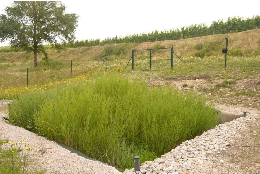
Figure 4.4. Overview of the horizontal subsurface flow constructed wetland.
