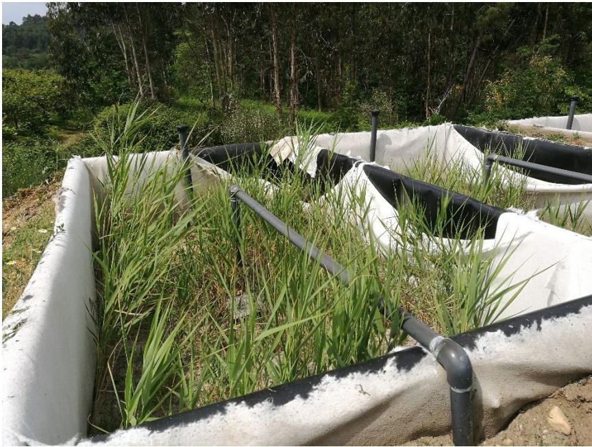
Figure 4.5. Overview of one of the sludge treatment wetlands.
