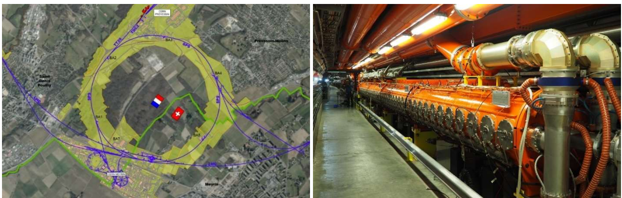
Fig. 6.1. Aerial view of the CERN SPS layout (left), and BA3 location detail in the tunnel hosting the SPS RF cavities (right).
