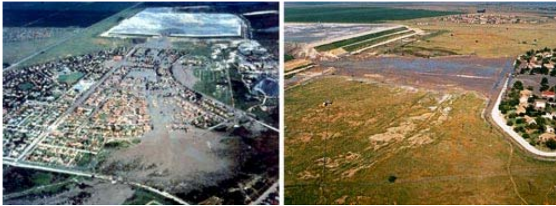
Figure 3.3. The failure of the slurry dam of Merriespruit due to flow liquefaction, Fourie et al. (2001).
