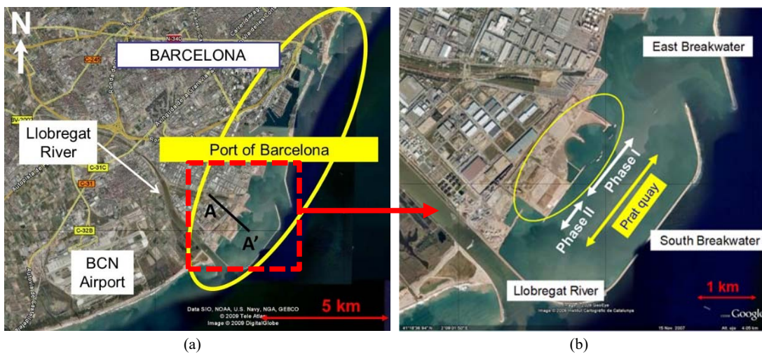
Figure 2.1. (a) Satellite image showing the location of the Barcelona Port. (b) Satellite image showing the Prat quay, the new breakwaters and the original and new Llobregat river mouth, source Google Maps.
