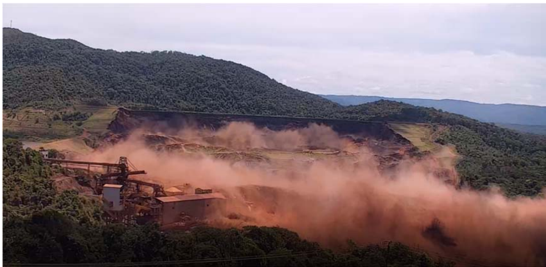
Figure 3.4. The failure of the tailings dam of Brumadinho due to flow liquefaction, source Youtube.
