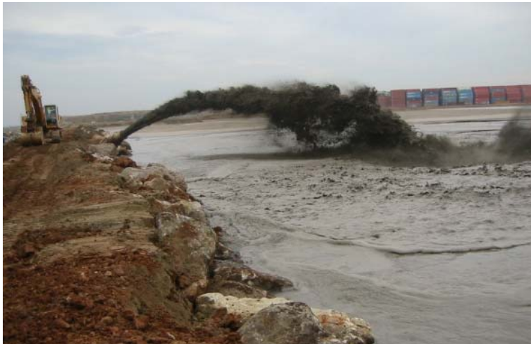
Figure 2.7. Rainbowing technique during construction, Prat quay.
