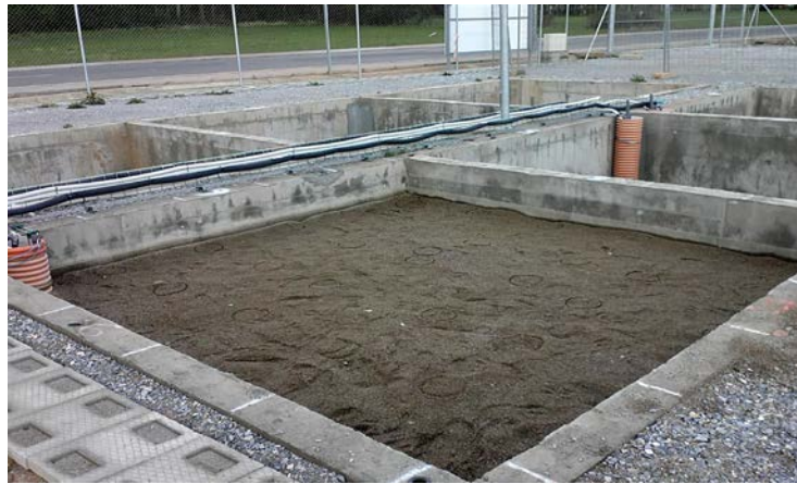
Figure 1. View of the experimental cell filled with gravel and coarse sand. The service well is located on the left corner.
