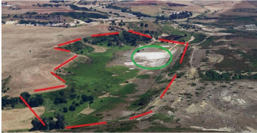
Figure 31. Aerial view of the Solfiorata di Pomezia, along its main axis. Picture taken from Google Maps. The red segments outline the area mined in the past for sulphur; the green circle shows an episodic flooded area.
