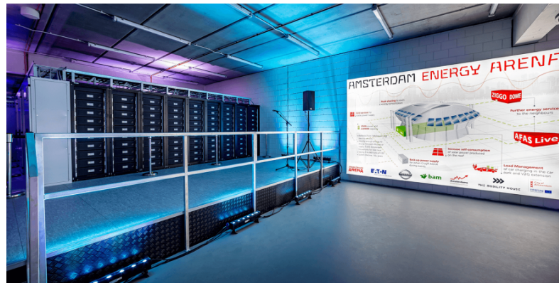
Figure 3.8: Second life LEAF batteries to power Amsterdam Arena
