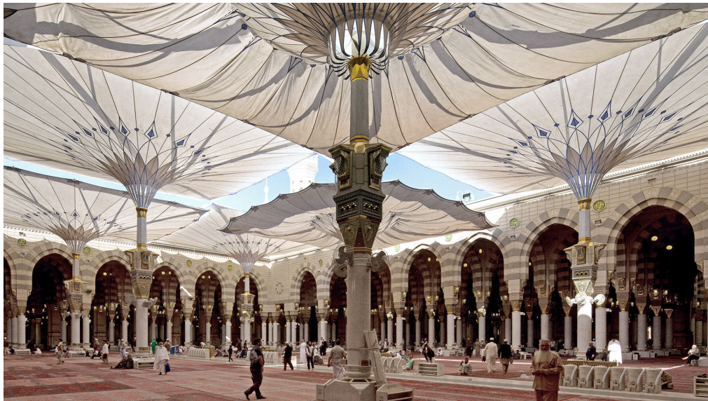
(b) Shading structure opened.
