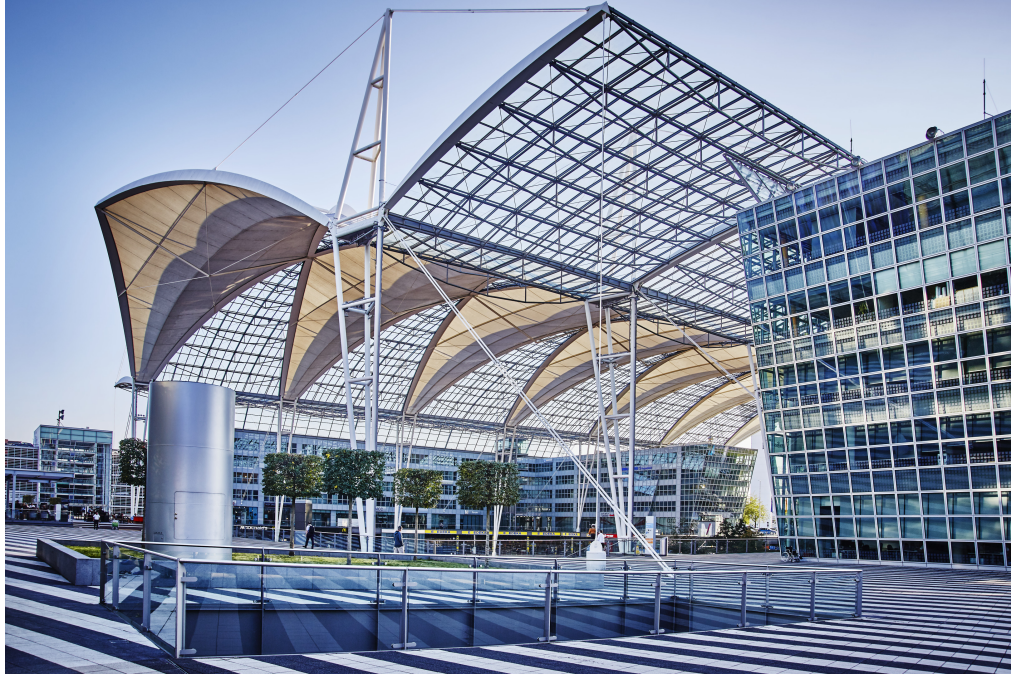
Figure 1.2: Textile roof cover in the airport of München.
