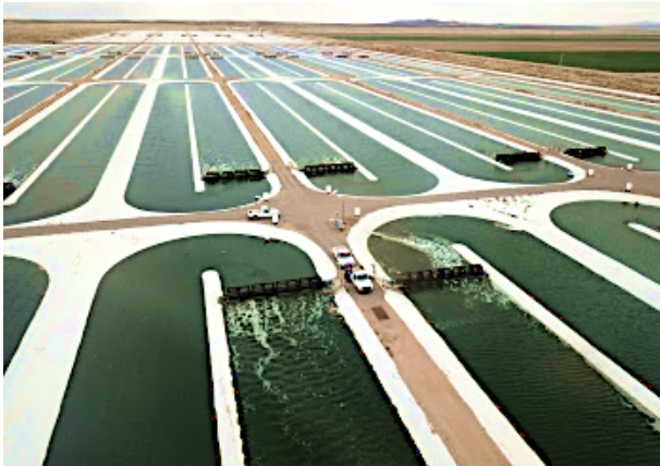
Figure 2-1. High rate algae ponds for microalgae biomass production from Qualitas Health (USA) (EERE, 2020).
