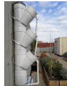
Figure 20 The WETWALL prototype – Fixation and allocation of the main structures (VF, HF and water reservoirs)
