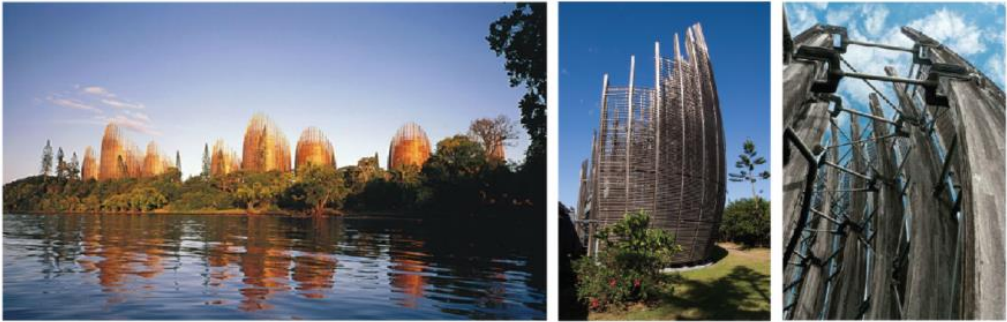
Figure 2.12. The Jean-Marie Tjibao Cultural Center and a focus on the metal anchors.
