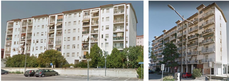
Figure 3.3. Views of the reference building. South-east (left) and north-west (right).
