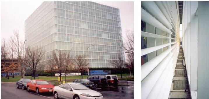
Figure 2.10. Main elevations of the Occidental Chemical Center and the focus on the cavity with the internal blinds.
