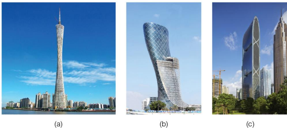
Figure 2.18. Pictures of the Canton Tower (a), the Capital Gate (b) and the Pearl River (c).
