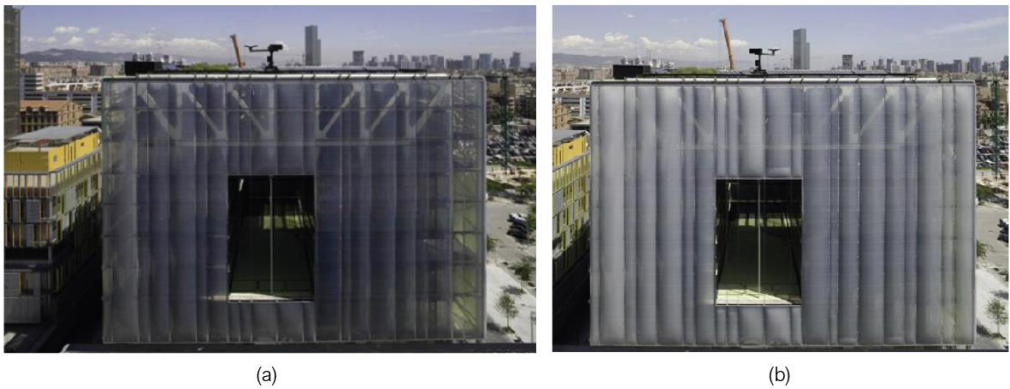
Figure 2.17. South-western elevation with the shading system off (a) and on (b).
