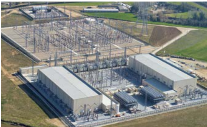
Fig. 1.8: INELFE project – Santa Llogaia substation in Spain (Courtesy of Siemens)
