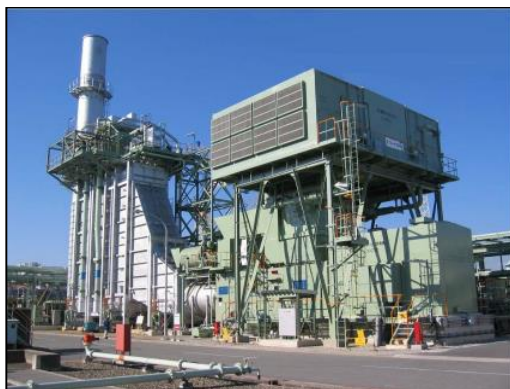
Figure 2.25. External view of the gas turbine and the HRSG installed at the Himeji LNG Terminal. Photograph of the Gas turbine intake air cooling system (Source: [192,197]) property of Osaka Gas Co. Ltd. and are included with permission. Schematic diagram redrawn and simplified from Ikeda [192].
