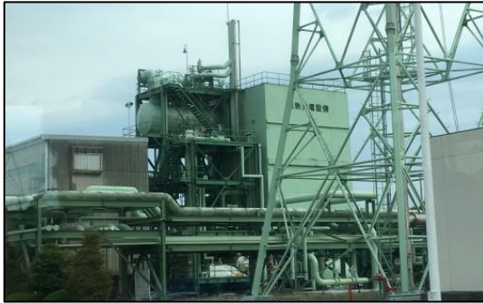
(a) Negishi Terminal (Tokyo Gas Co., Ltd.) Mixed fluid RC [100 t-LNG/h, Electric output: 4 MW]
