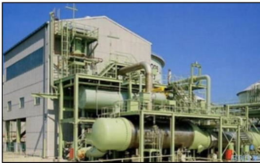
(b) Unit No. 2 Senboku II LNG Terminal (Osaka Gas Co. Ltd.) RC + DE unit [150 t-LNG/h, Electric output: 6 MW, Seawater usage: 6,000 t/h]
