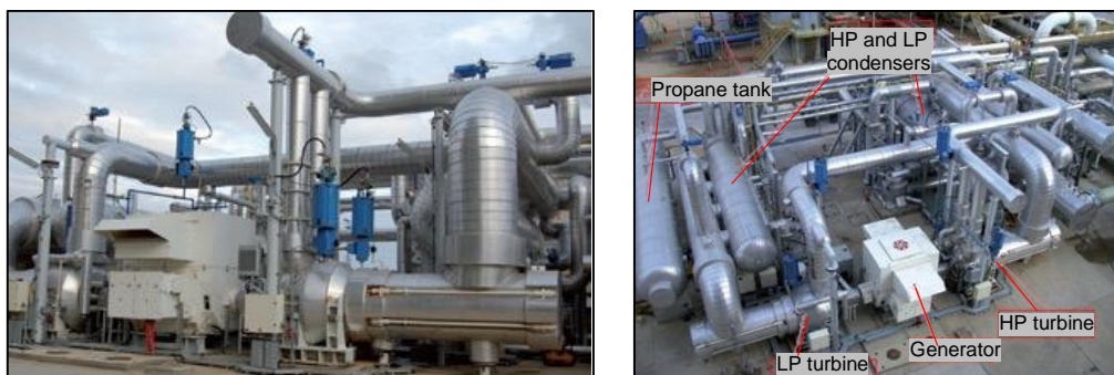
Figure 2.26. Photographs of the cryogenic power generation plant (Rankine cycle) installed in Huelva LNG Terminal and schematic diagram. Source: Photographs property of Enagás (included with permission) and obtained from [200]. Schematic diagram drawn according with the description of the system provided in [200].
