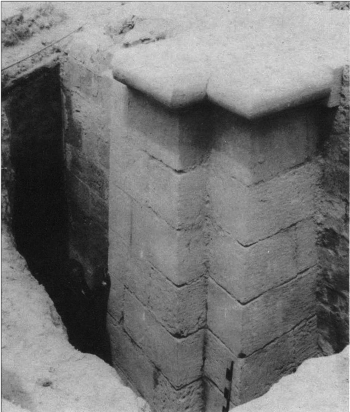
Fortification-point ( \gamma ). NW. corner of the Tulunid circuit (Site 4. Leclant 1979: Table II, Fig. 1)
