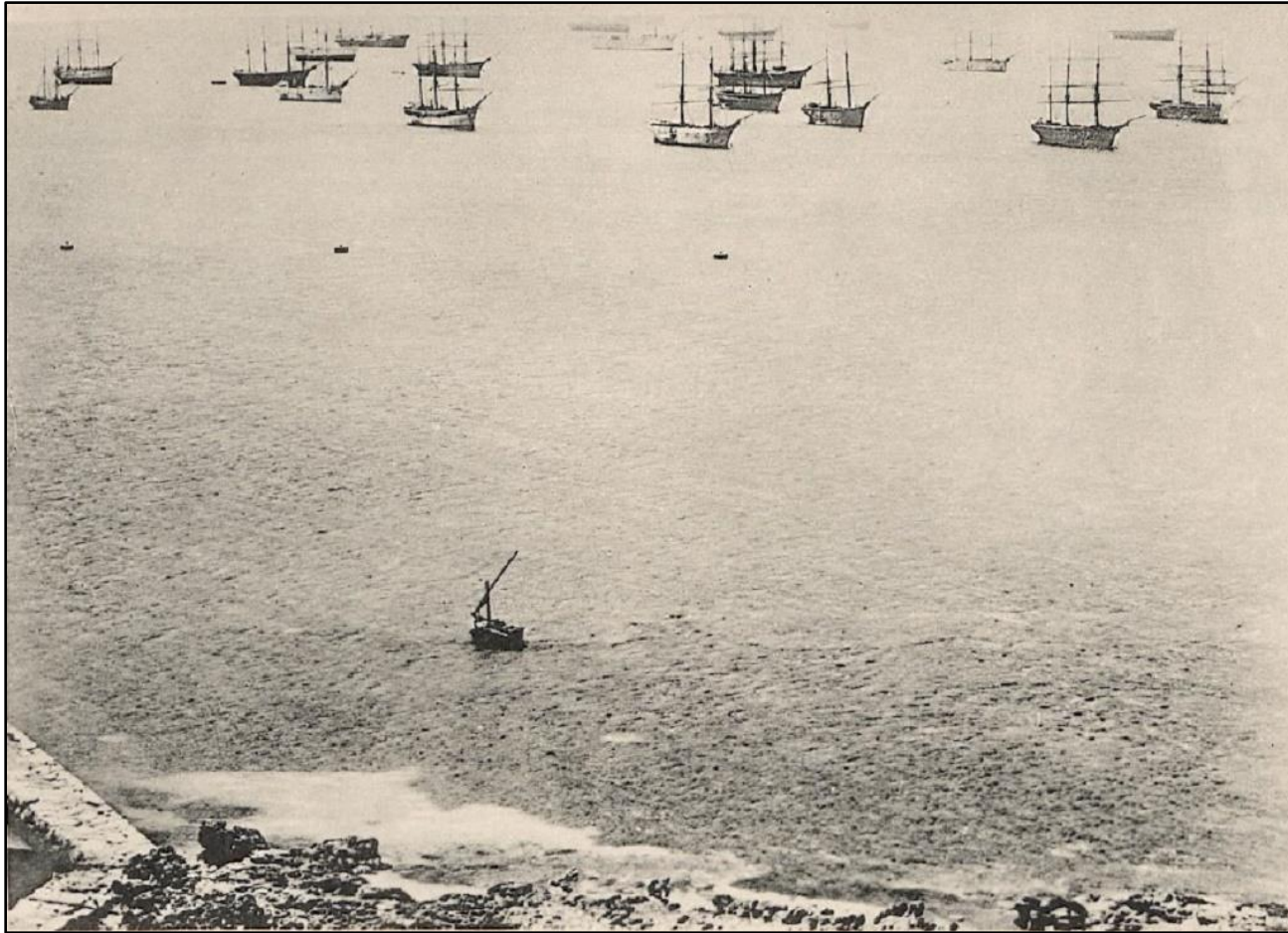
Submerged remnants of an ancient quay, seen from the Ras el-Tin lighthouse (Sec. 2.3.4. Jondet 1916: Fig. A)
