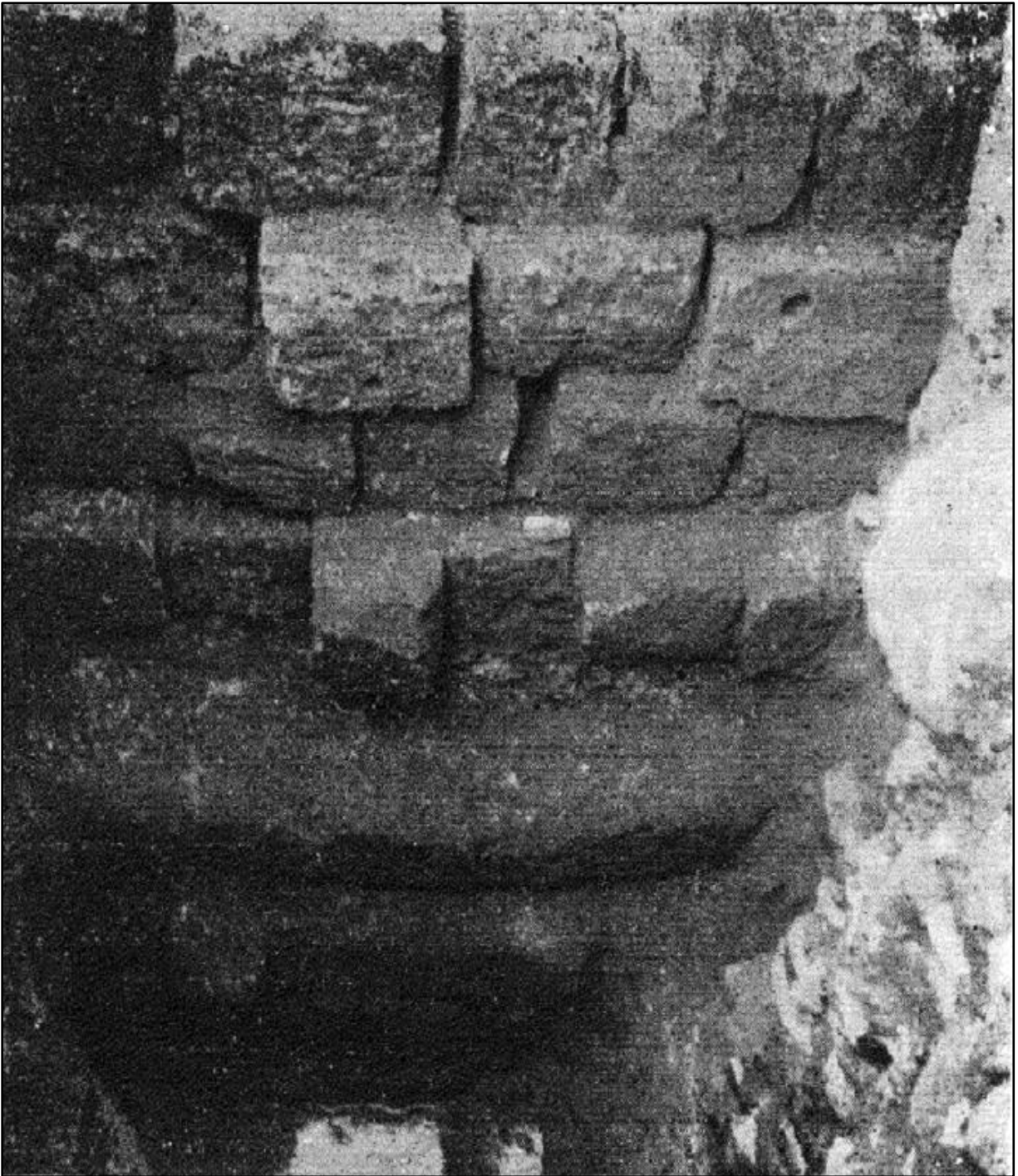
Cinema Amir, Kom el-Dikka. Main pit No. (11); foundations reaching groundwater-level (Site 17. Adriani 1956a: 4, Fig. 3)
