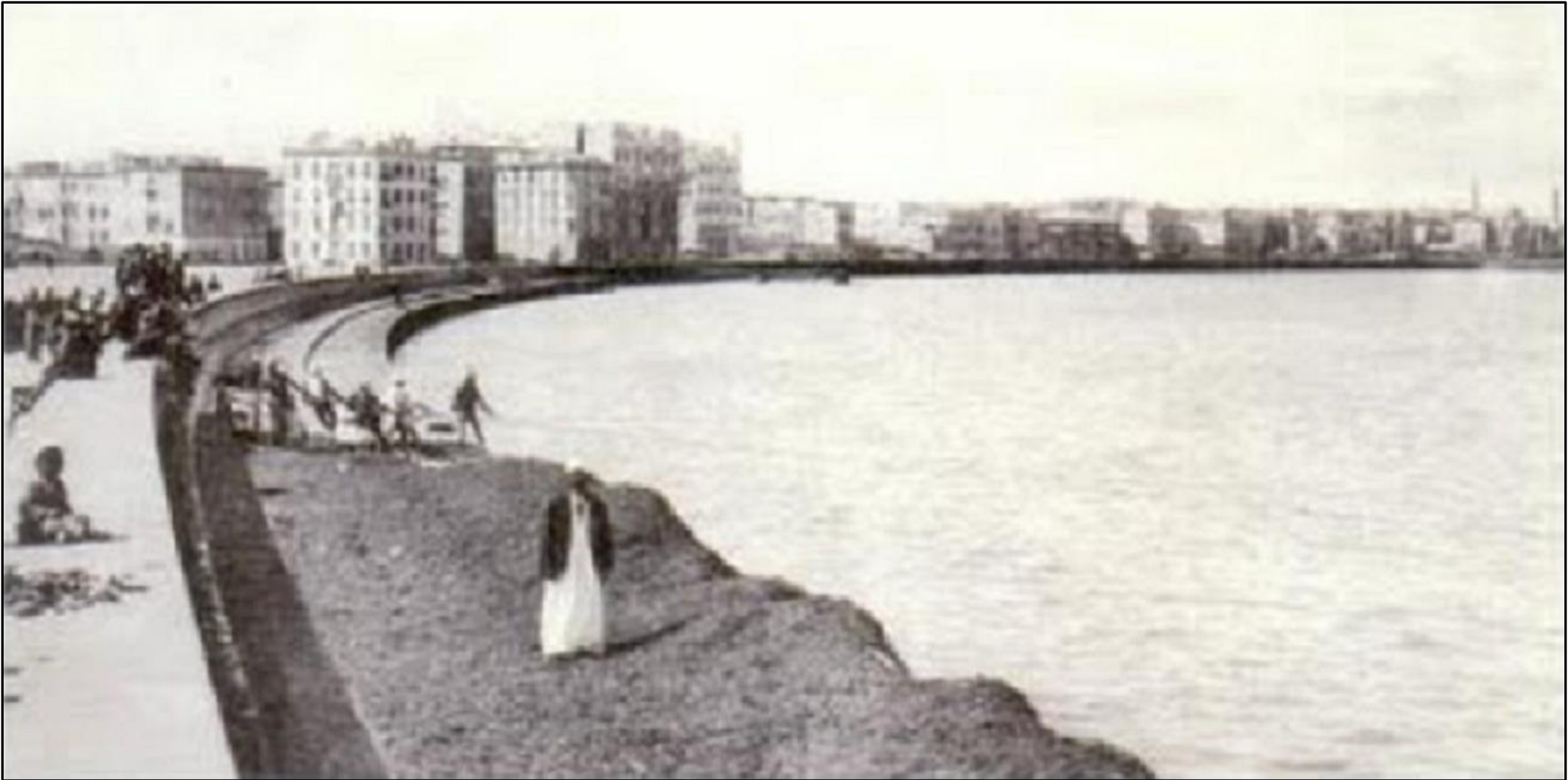
Construction of the Corniche (1906)
