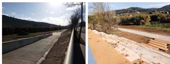
Fig. 2. Images of the renovated area of the Besòs Riverside Park: A) Renovated area of the Besòs Riverside Park, before and after the intervention; B) Provision of access to the riverbank.
