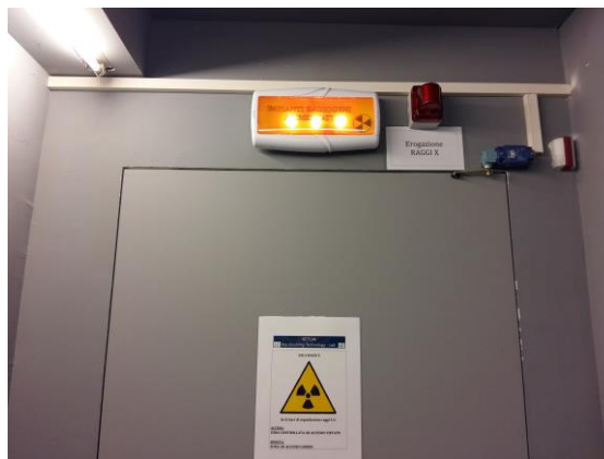
Figure 3.39 - External view of the experimental hall door. The device on the center signals that the X-ray tube receives the high voltage supply and is ready to be used, the red light on the right (light off) is a flashing one and indicates if the tube is on-going or not, the blue device on the right corner is the switch. The panel in the center contains the explanations of the flashing light.
