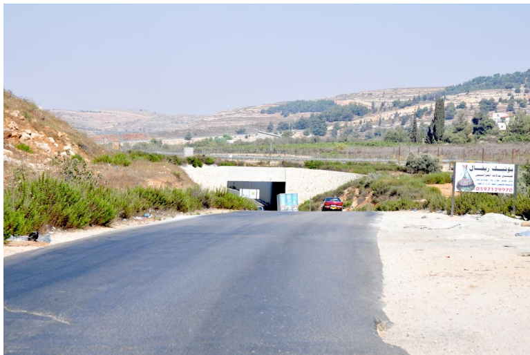
The tunnel road to Ramallah with the settler bypass road above it. Biddo, August 2013
