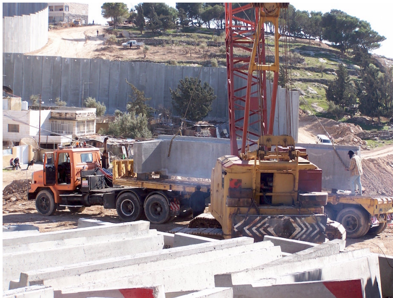
Wall in Abu Dis under construction. Abu Dis. January 2004.
