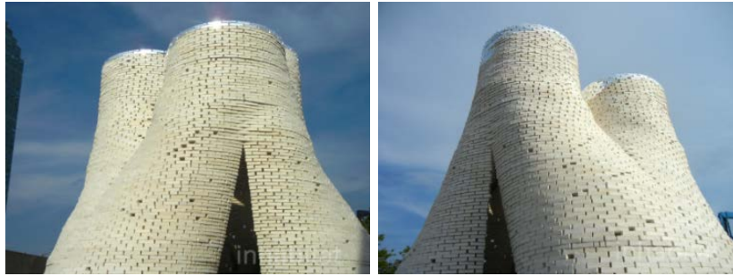
Image [26, 27]. The complete built Hy-fi towers proving the potentials of mycelium composite panels as a temporal building materials.
