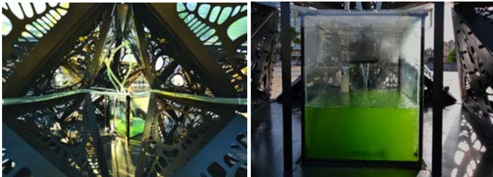
Image. [59, 60]. Left, interior view of the device showing the assembly of tubes and its relation with structural design using perforated metal to allow natural lighting for the container fixed inside the perforated panels ETFE cladding system of the device. Right, the micro algae container containing the nutrient medium. Ecologic Studio.
