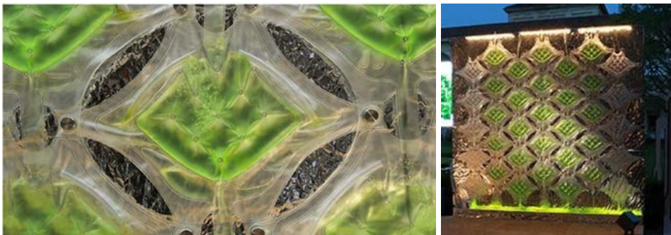
Image [34]. The single micro algae biofilm unite. Right the cladding system. Ecologic Studio
