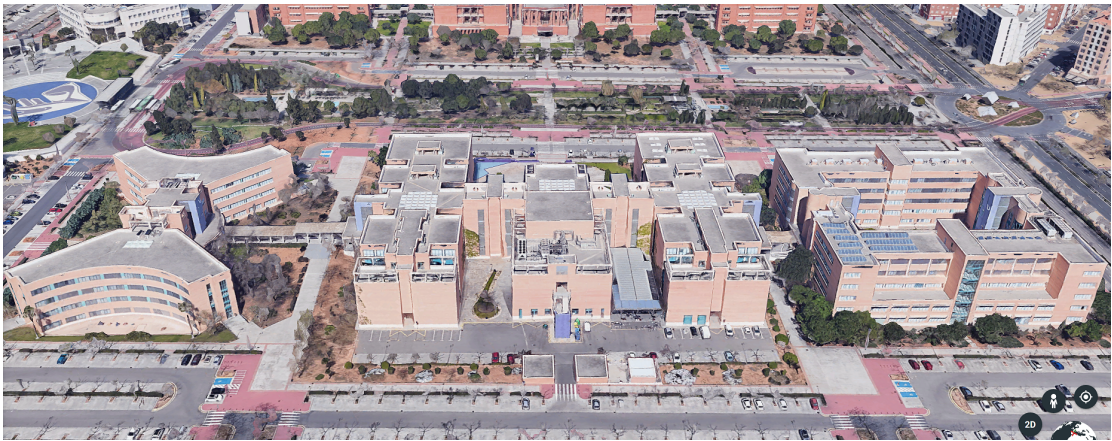
Figure 6.4: 3D areal view, from Google Earth, of the three buildings considered in this section’s experiments. From left to right, the buildings are identified as TI, TD and TC.
