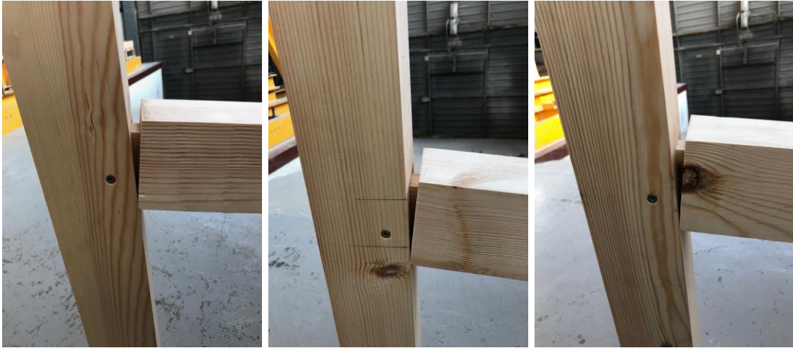
Figure 4. 72: Failure pattern of three specimens under cyclic loading
