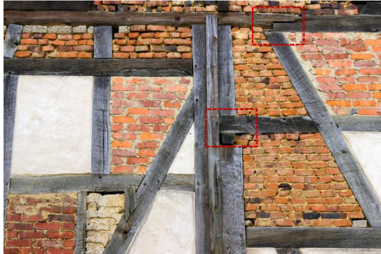
Figure 2. 4: Timber joints in frame (Turkish Timber Association, 2018)
