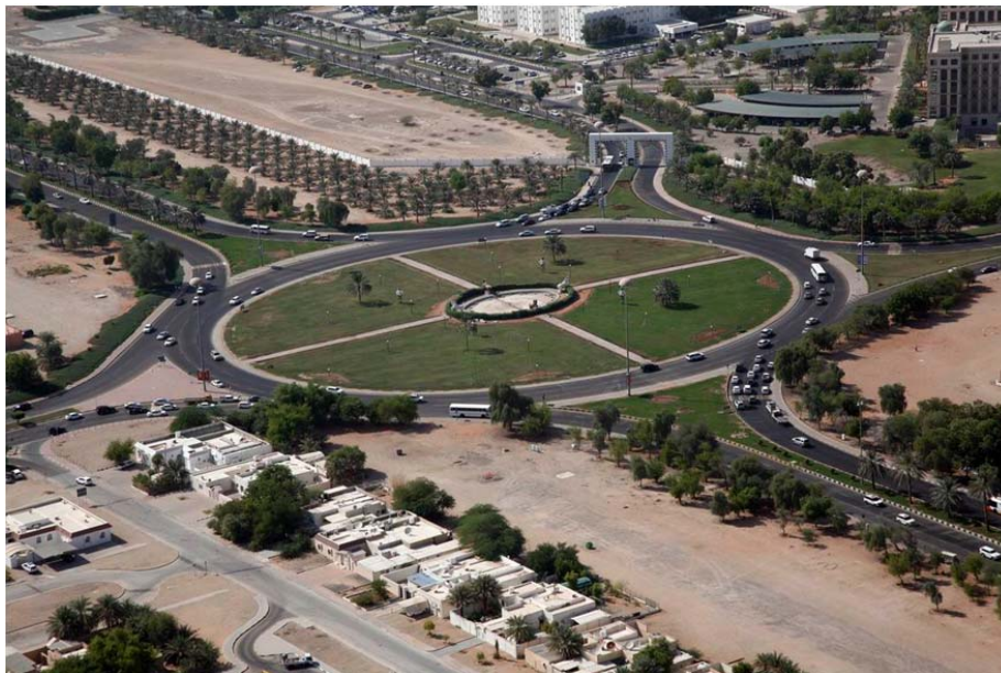
Photograph 2.3. Example of planned green roundabout. Source: Al Ain Municipality, 2009.
