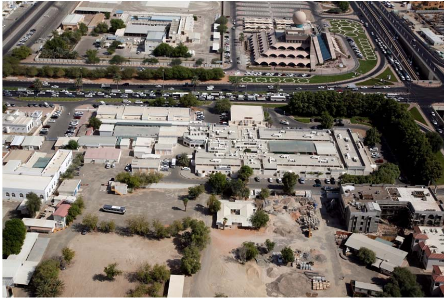
Photograph 2.9. Oasis Hospital in Al Mutawa'a. Source: Al Ain Municipality, 2009.
