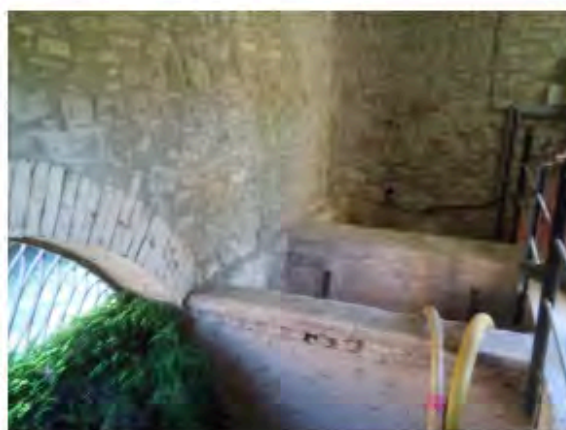
FIG. 4. Inside the hydrometric module building.
