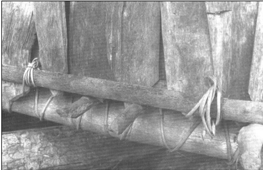
Fig.169: Darai house (Indonesia). The base plane and vertical plane elements are connected using ropes made of natural fibres (Pétrequin 1988).
