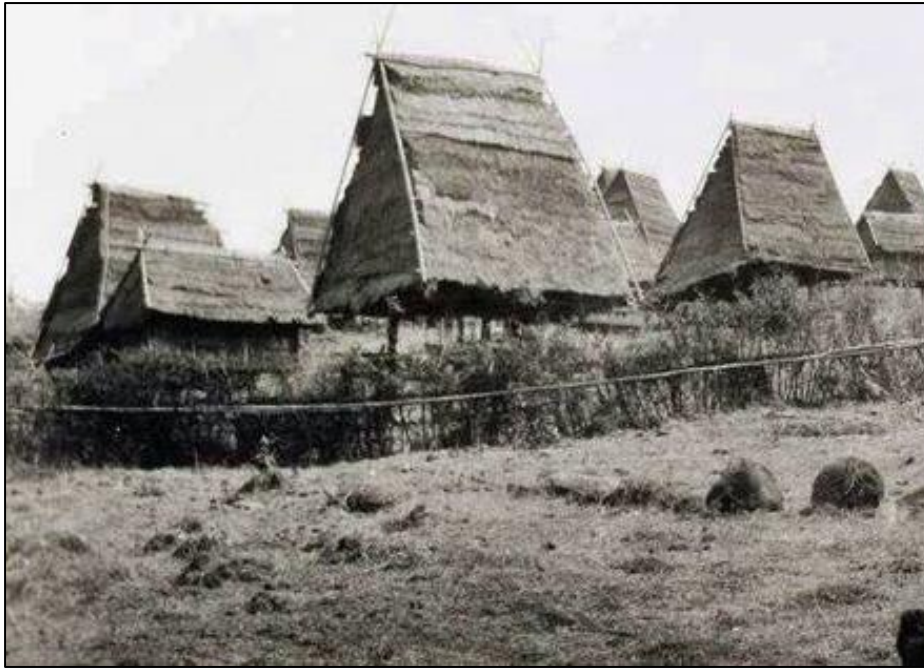
Fig.164: Sumbawa houses (Indonesia): these houses usually have no openings except for the frontal door. In case of necessity, holes can be easily obtained piercing the walls made of vegetal elements ( https://alanmalingi.wordpress.com ).
