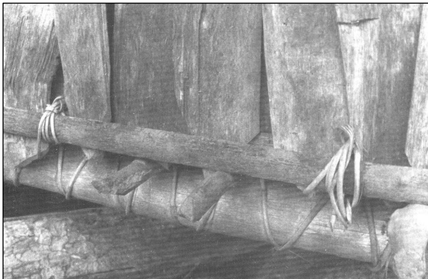
Fig.115: Darai house (Indonesia). The base plane and vertical plane elements are connected using ropes made of natural fibres (Pétrequin 1988).
