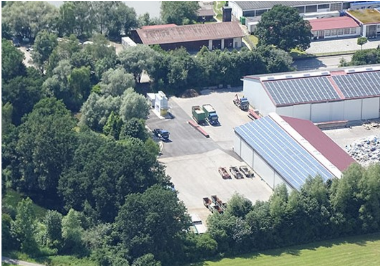
Figure 3.5: Aerial photo of the SmartPowerFlow BSS prototype.
