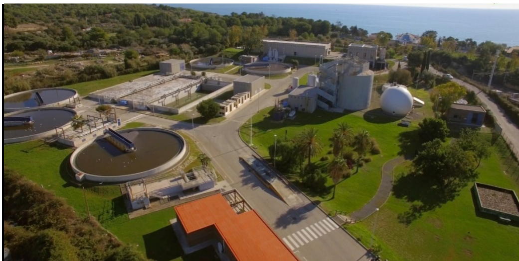
Figure 2.2. Aerial view of Vilanova WWTP, location of the pilot plant.
