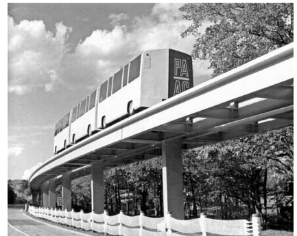
Figuras A5.42 y A5.43 – El Transit Express-way de la Westinhouse - "Skybus". Fuente: http://www.brooklineconnection.com/history/Facts/Skybus.html
