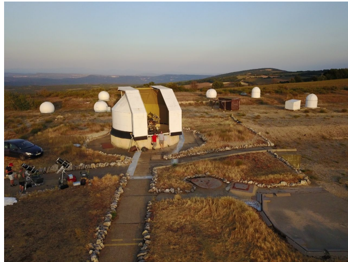
Figure 5.1.5: Aerial view of the refurbished dome at Sirene's Observatory, France.
