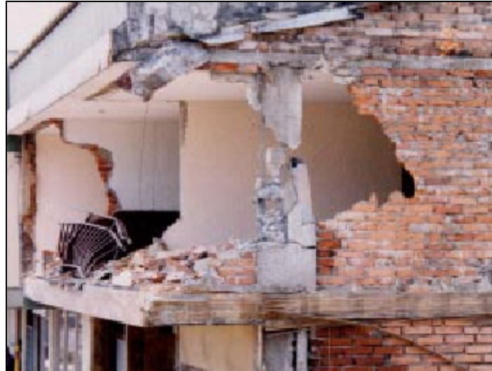
Picture 7: Damage to a RC a column, building in Armenia, Colombia [Yoshimura et. al, 1999].
