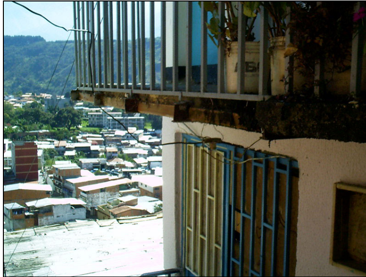
Picture 3: Detail of a slab (balcony in a sloped site building).
