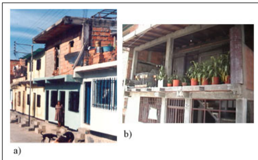
Picture 16: Roof Types in Barrios. a) Slab roof in one or more levels, and metal sheeting roof in two levels. b) Tile roofing supported over wooden deck and “I” shaped steel beams.
