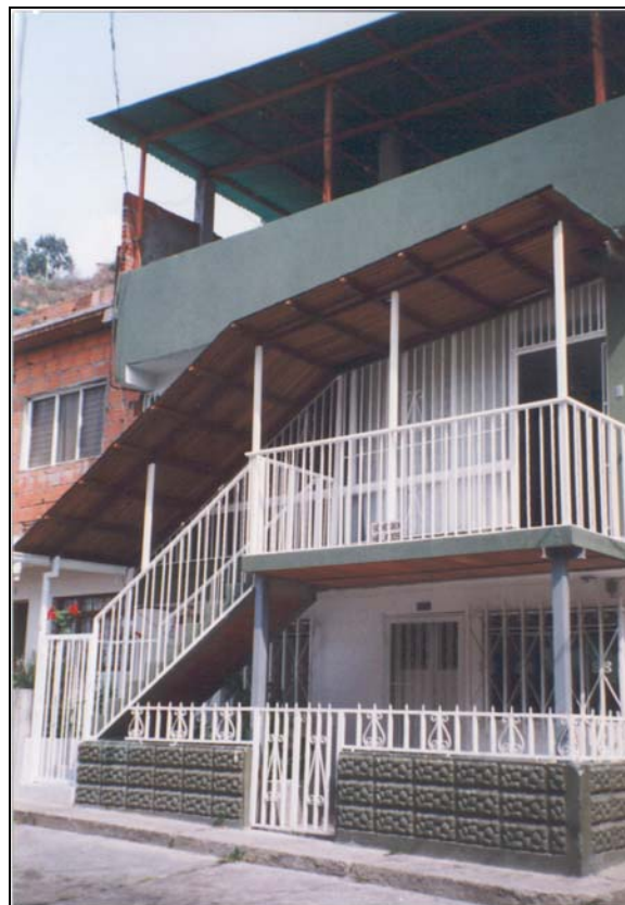
Picture 4: Stair in the front of a building.
