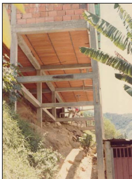
Picture 17: High-slope site for housing unit, structural members are observed in different lengths, with low-ductility elements in the middle structural axis, see columns over the foundations.
