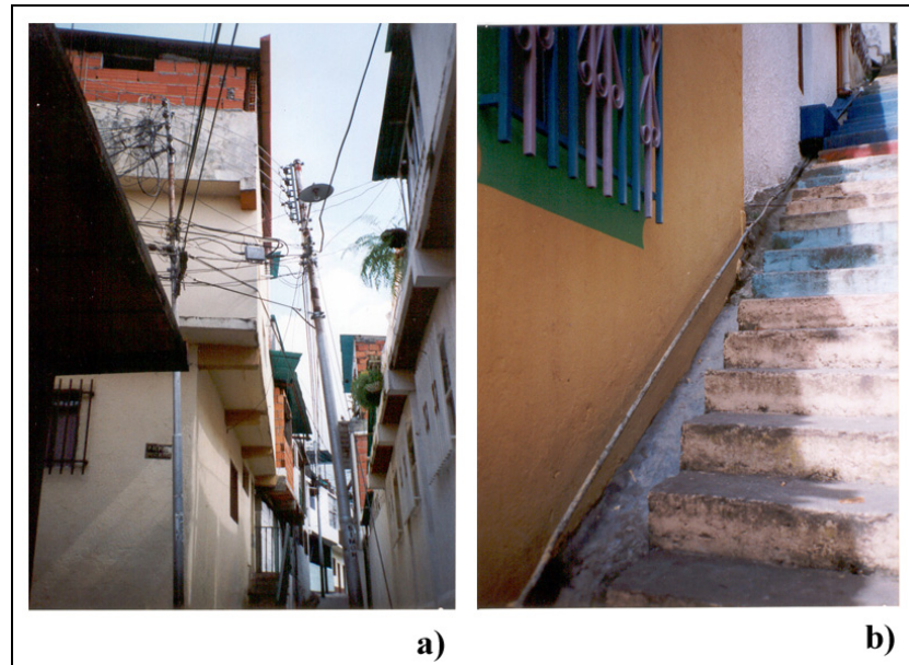
Picture 1: Electricity and water supply in La Milagrosa Barrio.
