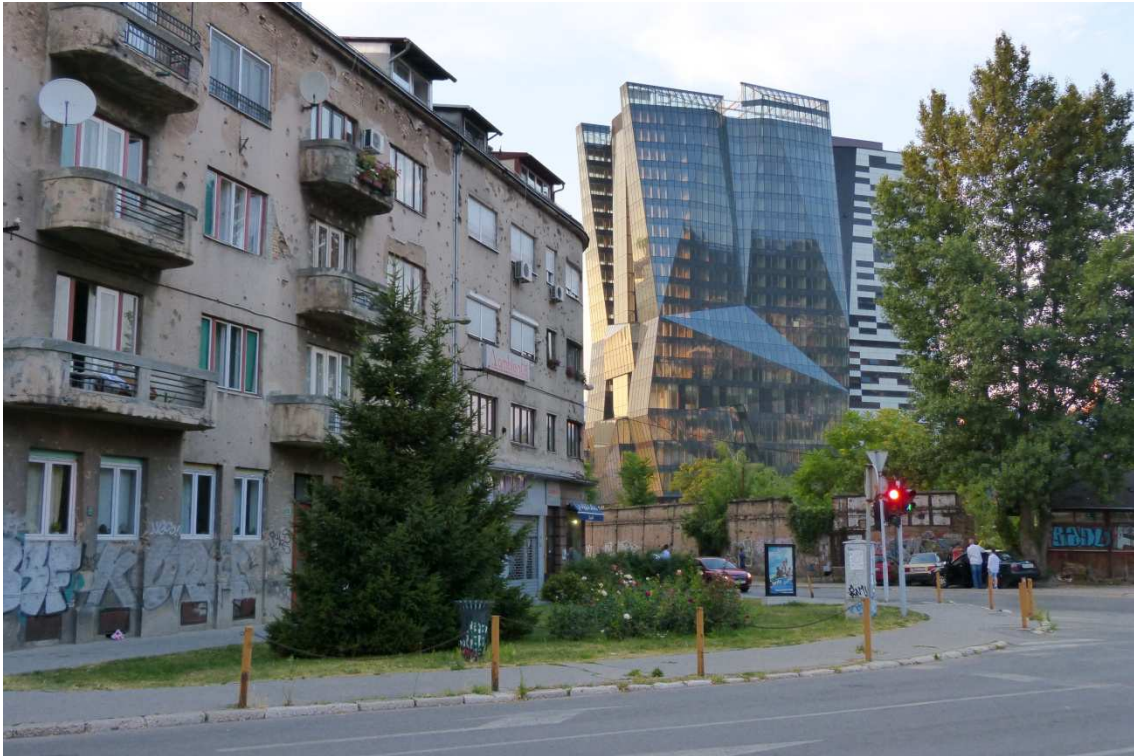
Figure 13. Redevelopment of the Marijin Dvor area, with the Sarajevo City Center. Author's picture.
