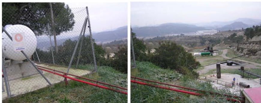
Figure 2.4. View of the pressurized vessel containing liquefied propane (approximate conditions: temperature, 25°C; equilibrium vapour pressure, 9.5 bar).
