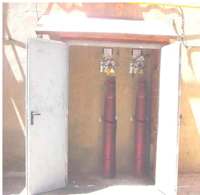
Figure 5-2: Explosion-proof compartment for gases.
