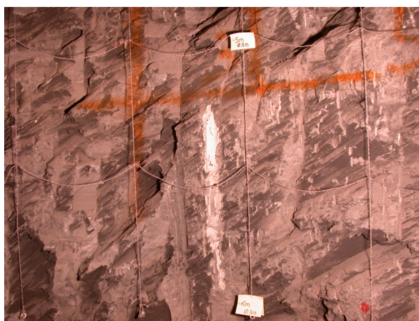
Figure 6.4: Cross-anisotropic Opalinus clay rock in the wall of the excavation, during the dismantling of the HE experiment.
