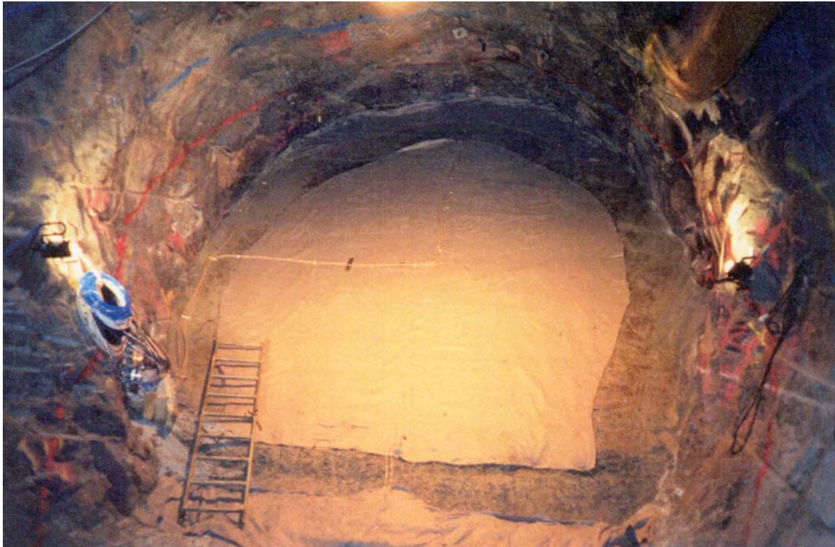
Figure 2.16: Detail of three permeable mats placed after the compaction of one of the layers (Gunnarsson et al. 2001).
