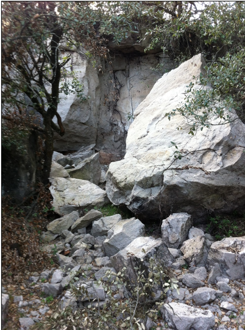
Figure 3: Picture of the Lluçà rockfall case inventoried. A huge block conserve the main part of the total rock mass detached.
