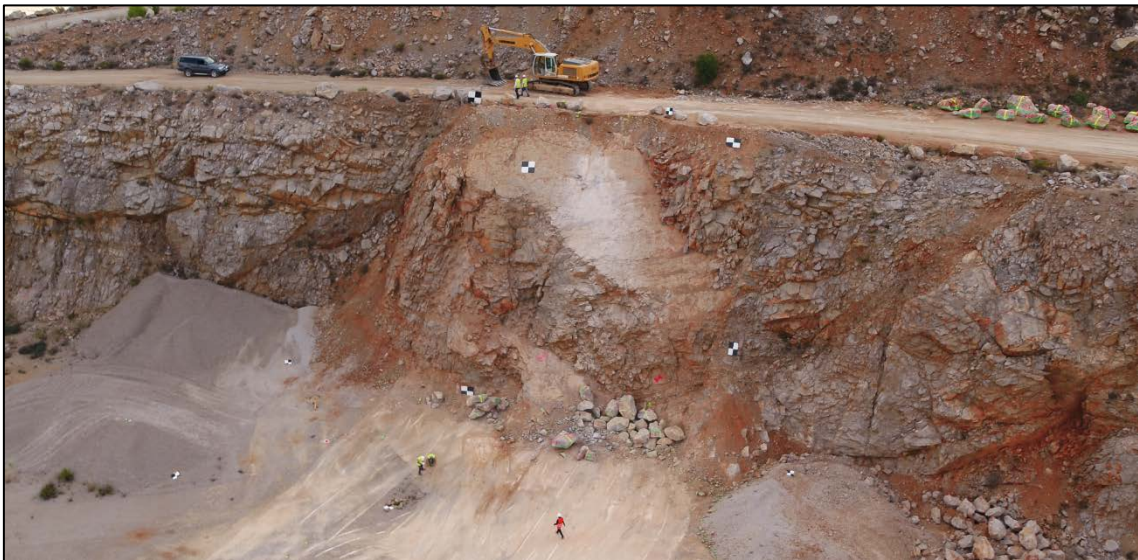
Figure 1: Picture of real-scale fragmentation test on a quarry (Test 4).
