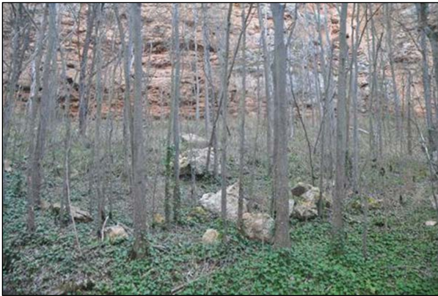
Figure 11. Blocks resting at the bottom of cliff B. These blocks were removed from the cliff during the scaling works carried out in 2015 and are used to calibrate the RockGIS model.
