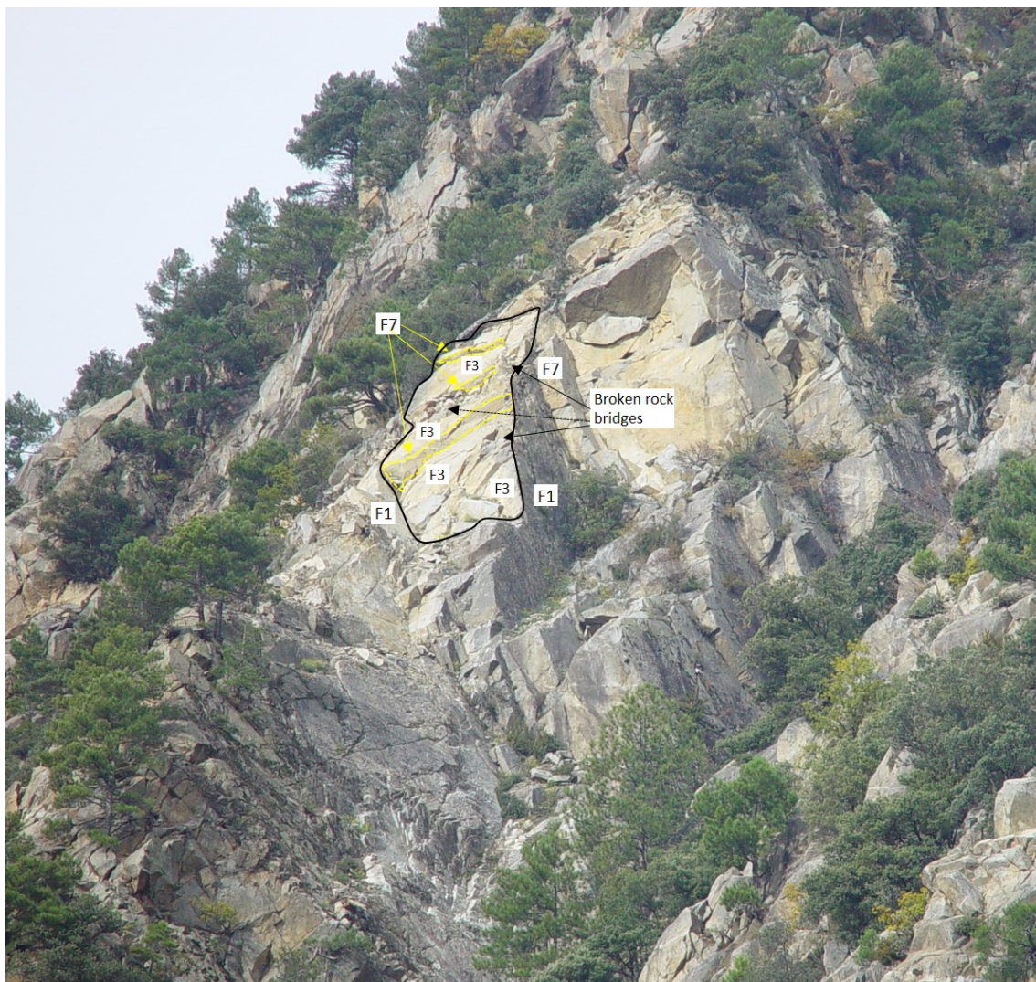
Figure 15. Rockfall scar of April 20th, 2008. The failure developed over several adjacent down-dipping planes (F3) generating a stepped sliding surface (black solid line). Steps are formed F7 planes (yellow dashed polygons) and broken rock bridges. The failure is bounded laterally by planes of F1 set.
