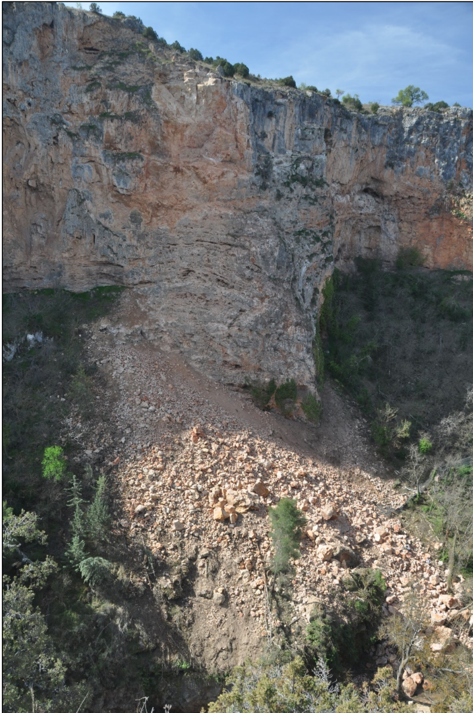
Figure 8. left: general view of the rockfall event of February 2017.
