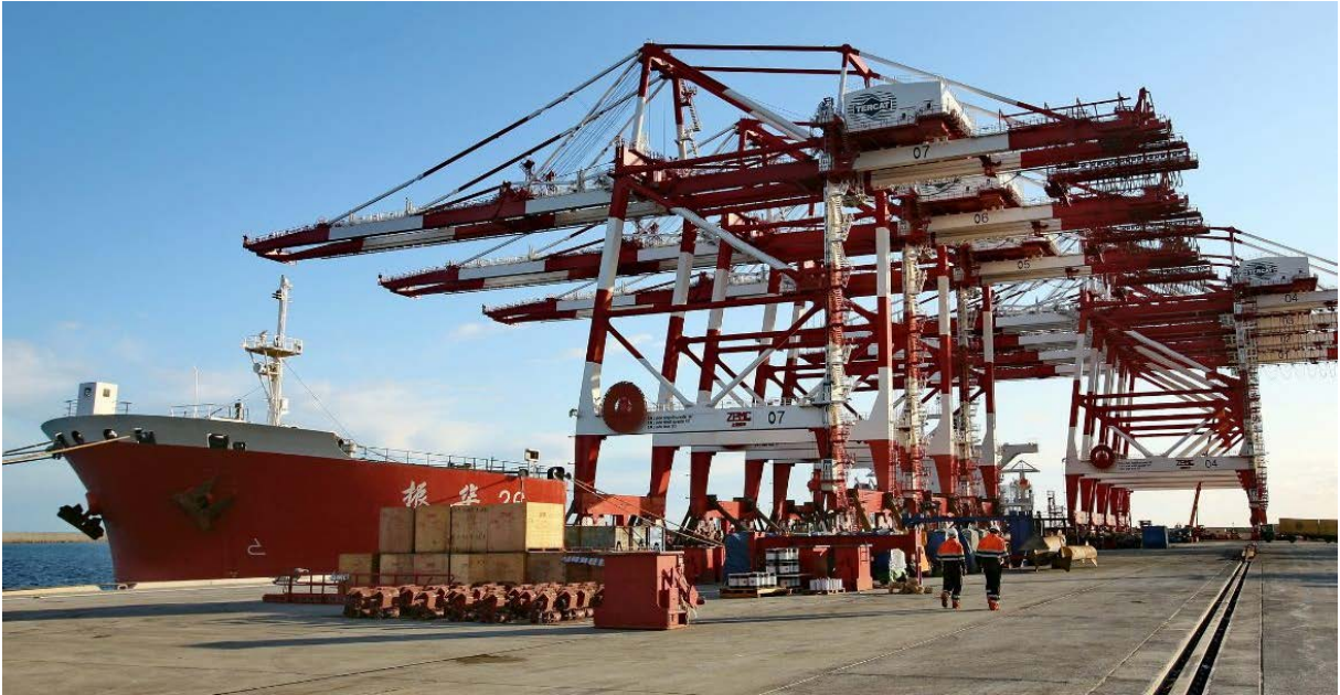
Figure 19. STS cranes at quayside.
