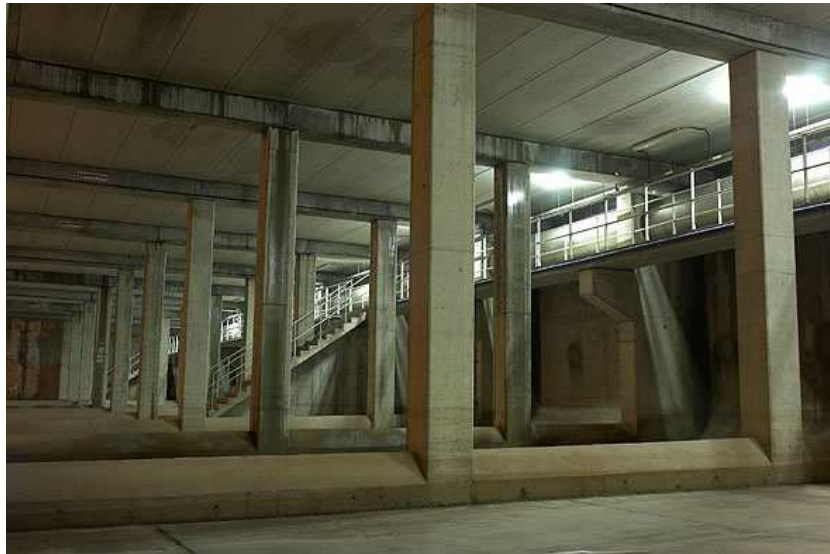
Figure 2.3: Retention tank (inner face). Taken from [CLA05].
