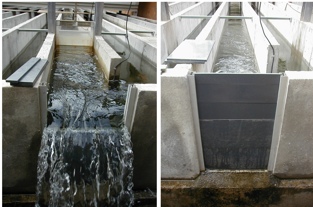
(a) Opened weir
