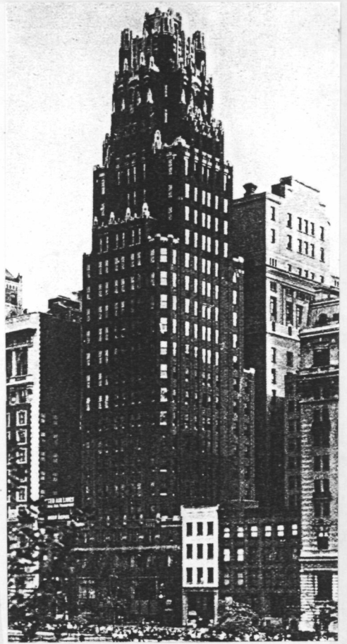
AMERICAN RADIATOR BUILDING N.Y. 1924.
